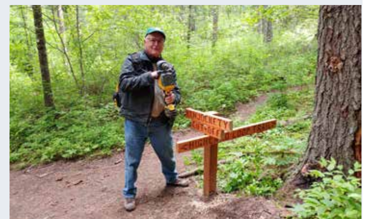
Below: Dave installing new directional and trail signs at Idler's Rest.
